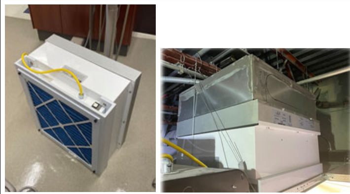
Figure 6. Left: Reverse flow HEPA scrubber; right: HEPA scrubber mounted above the ceiling grid for DTR.
